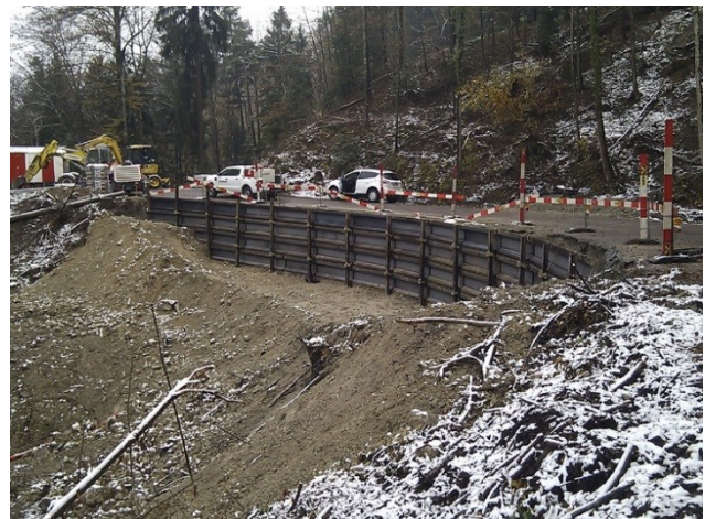
Illustration 35 Palissade terminée (Ribbert AG)
